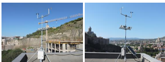
Figure 4. Sensor M187, Its surrounding area and construction
